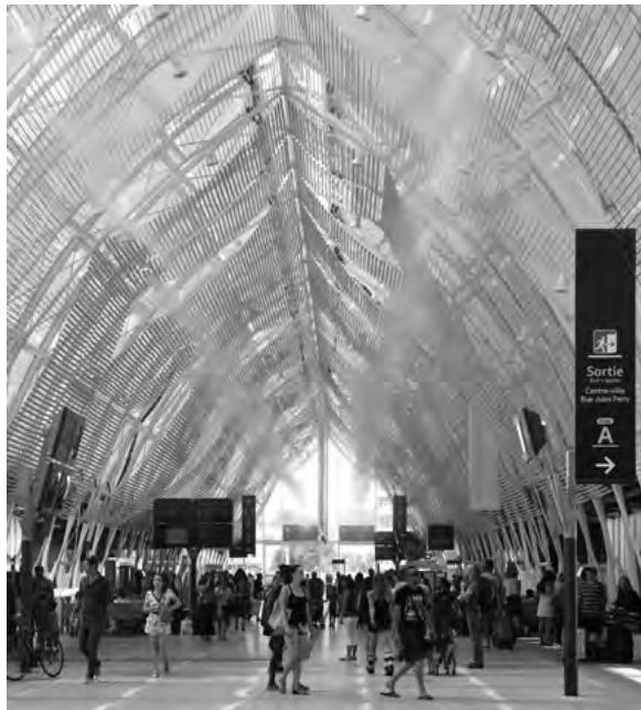
Mist cooling system in Montpellier Saint-Roch station.
