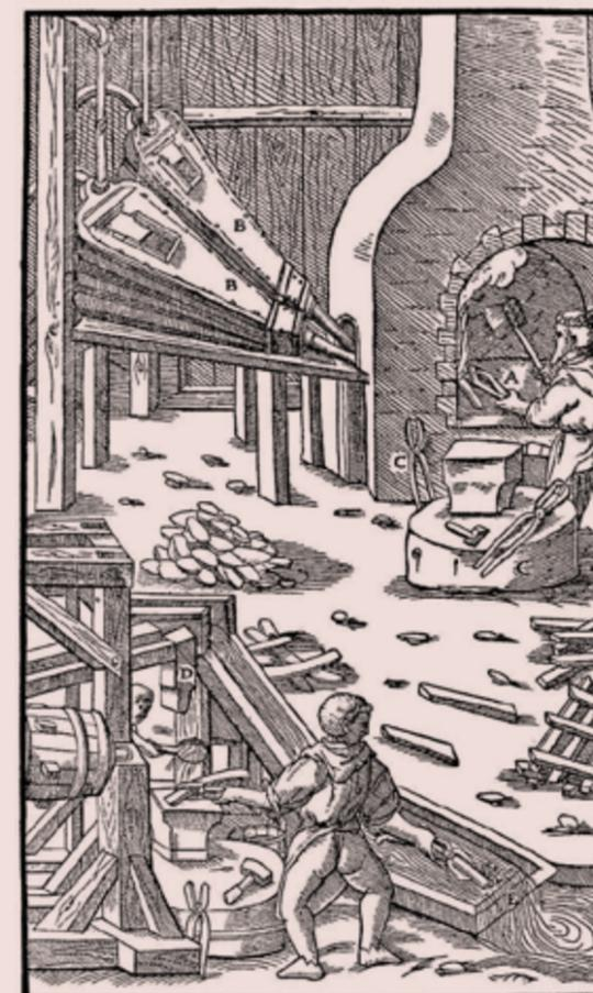
A—FORGE. B—BELLOW. C—TONGS. D—HAMMER. E—COLD STREAM.
