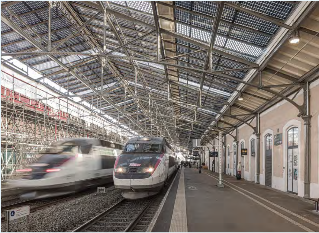
Grand Passenger Hall solar-powered in Angoulême, France
