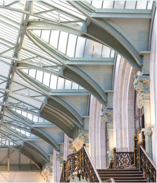
Renovation of the Small Passenger Hall in Paris Lyon train station, France
