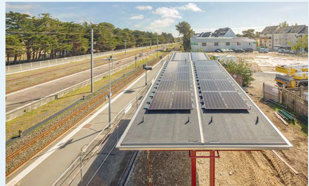
The new solar shelter developed by AREP, combining frugality, aesthetics, and ease of operation, France
