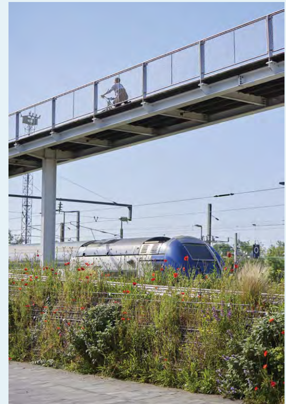
Footbridge for cyclists and pedestrians in Béthune, France
